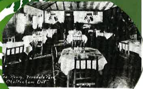
Tearoom, Ferndale Pavilion, 1931
